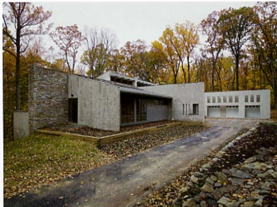
The conceptual design for the striking Neeff residence began with the 130-foot wall of stonework that serves as both the center support and the main focal point of the home. The wall (seen at left) extends the full length of the structure.
